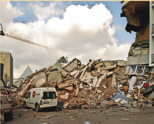
Figure 3: The collapsed Cologne city archive. Photo courtesy of Frank Domahs, Cologne, 2009
